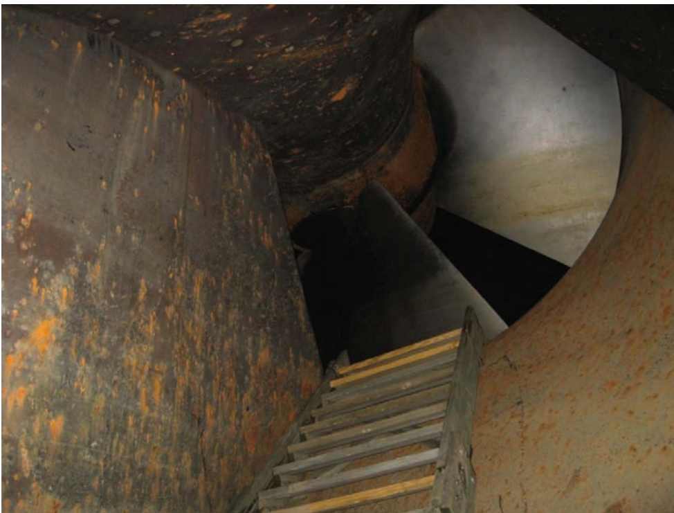
Photograph 5: Turbine Runner Blades
